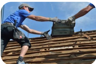
Picture 1: John, roofer (source: AMH)
